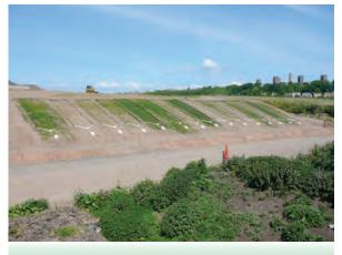
Figure 3 WRAP slope at Riverside, showing amendment with quality green compost enhancing grass establishment.
