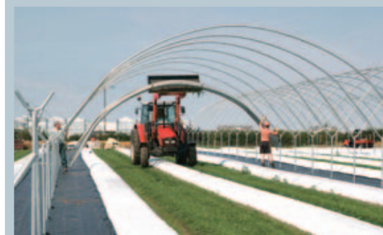
Construction of Spanish tunnels
